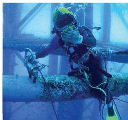
Lastek 1000 cutting all metals without compressed air
