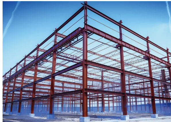
Steel structure industry
