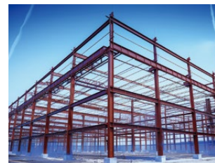
Steel structure industry
